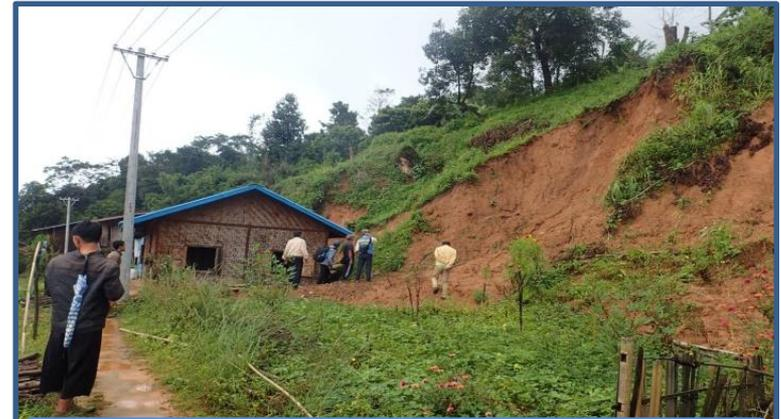
5. Poor Drainage System (Increasing Pore Water Pressure)
