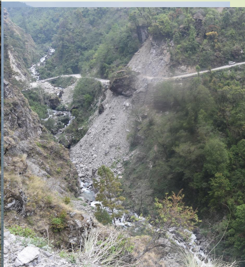
Khopang cliff (rock fall), and debris slide, North of Dhunche, 2018.
