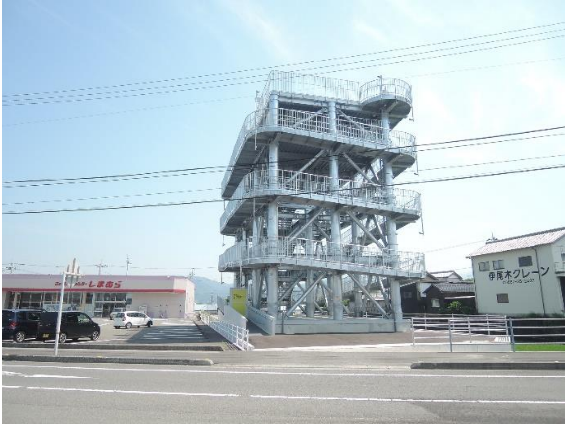
Tsunami tower at Aki.
